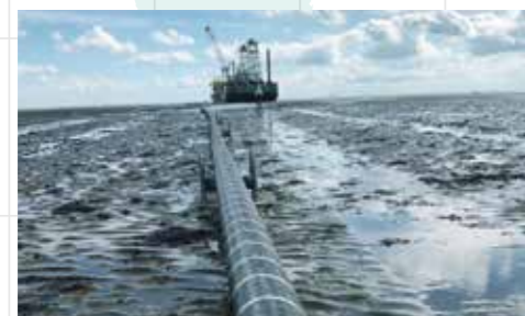
Submarine cable being installed
